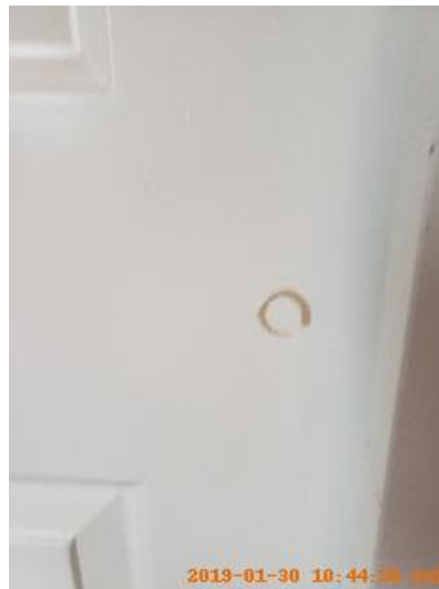
Closet/Door/Track/Shelving Taken on: 2019-01-30 10:44:36 Taken at: 43.70715948, -116.62555005 Image
