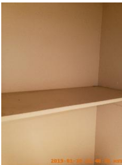
Cabinet/Counter/Shelving Taken on: 2019-01-30 11:48:36 Taken at: 43.70715978, -116.62564899 Image
