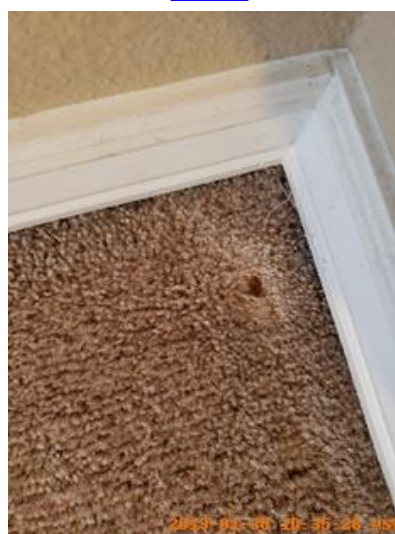
Flooring/Baseboard Taken on: 2019-01-30 10:35:28 Taken at: 43.70722721, -116.62559094 Image
