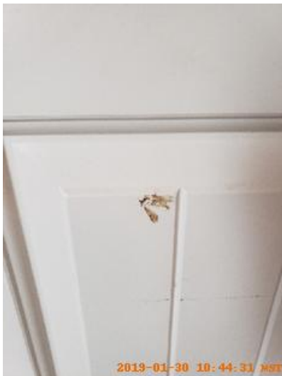
Closet/Door/Track/Shelving Taken on: 2019-01-30 10:44:31 Taken at: 43.70716177, -116.62555097 Image
