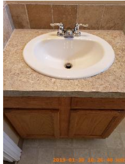
Cabinet/Counter/Shelving Taken on: 2019-01-30 10:26:40 Taken at: 43.70715212, -116.62553689 Image
