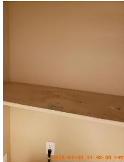
Cabinet/Counter/Shelving Taken on: 2019-01-30 11:48:30 Taken at: 43.70716086, -116.62565149 Image
