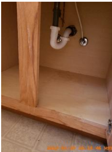
Cabinet/Counter/Shelving Taken on: 2019-01-30 10:18:46 Taken at: 43.70718751, -116.62555758 Image
