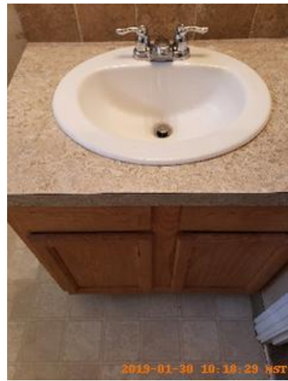
Cabinet/Counter/Shelving Taken on: 2019-01-30 10:18:29 Taken at: 43.70718751, -116.62555758 Image
