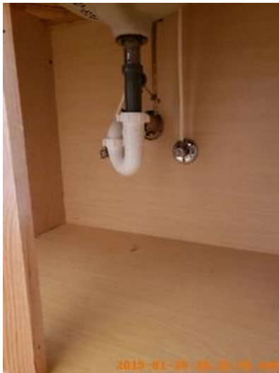
Cabinet/Counter/Shelving Taken on: 2019-01-30 10:26:56 Taken at: 43.70706812, -116.62548941 Image
