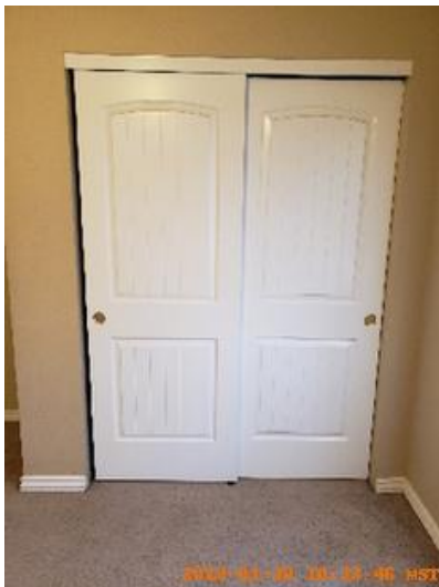
Closet/Door/Track/Shelving Taken on: 2019-01-30 10:33:46 Taken at: 43.70717169, -116.62558597 Image
