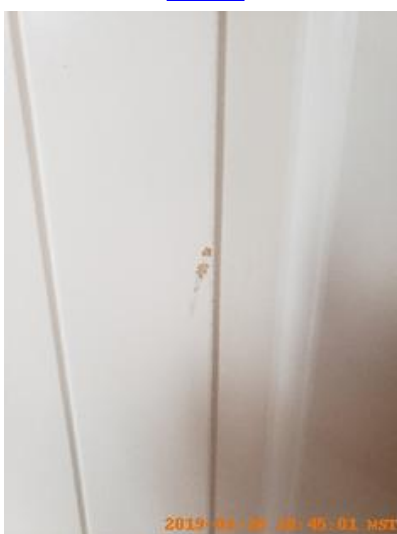
Closet/Door/Track/Shelving Taken on: 2019-01-30 10:45:01 Taken at: 43.70715992, -116.62555051 Image
