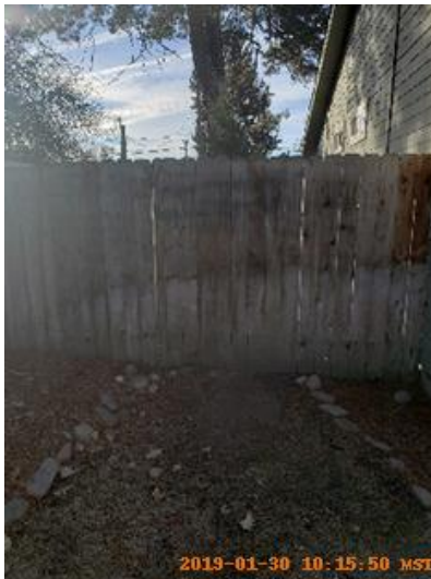
Fence/Gate Taken on: 2019-01-30 10:15:50 Taken at: 43.70725805, -116.62562741 Image
