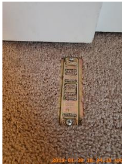
Closet/Door/Track/Shelving Taken on: 2019-01-30 10:34:15 Taken at: 43.70721527, -116.62556669 Image
