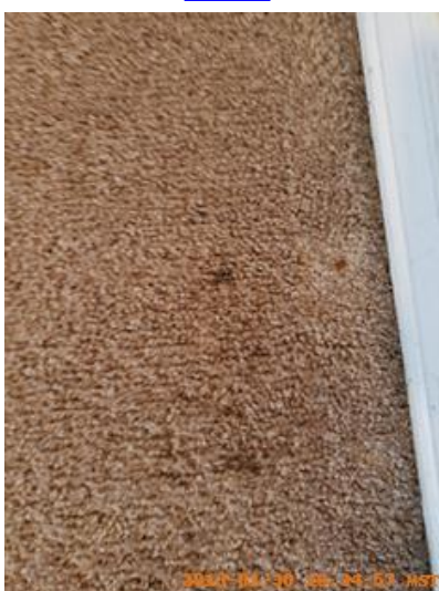
Flooring/Baseboard Taken on: 2019-01-30 10:34:57 Taken at: 43.70722721, -116.62559094 Image
