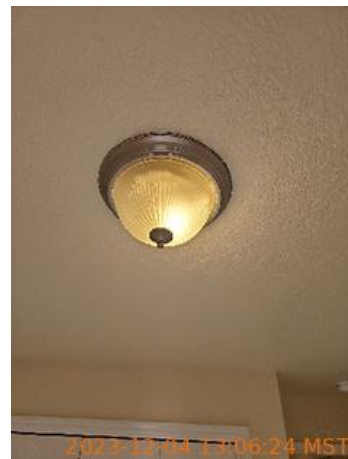
Light Fixture/Fan 📅 2023-12-04 13:06:24 📍 43.6959292, -116.4917973 🖼️ Image
