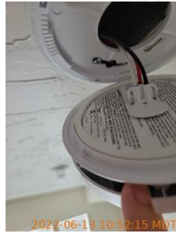
Smoke / CO detector
