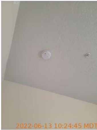
Smoke / CO detector
