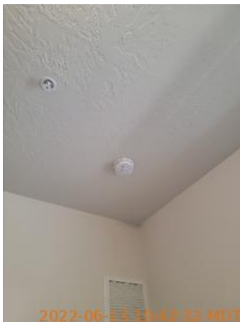
Smoke / CO detector
