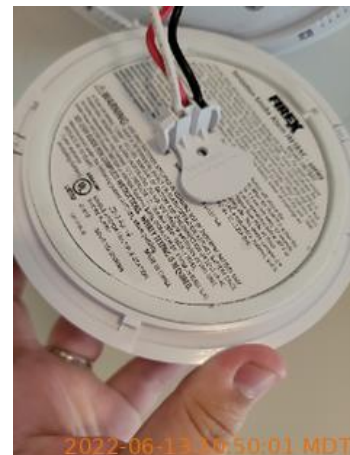
Smoke / CO detector
