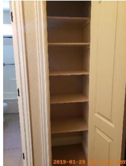
Closet/Cabinet Taken on: 2019-01-29 13:13:41 Taken at: 43.56529137, -116.60389785 Image
