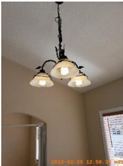
Light Fixture/Fan Taken on: 2019-01-29 12:58:36 Taken at: 43.56527021, -116.60379613 Image
