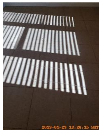
Flooring/Baseboard Taken on: 2019-01-29 13:26:15 Taken at: 43.56526833, -116.60381408 Image
