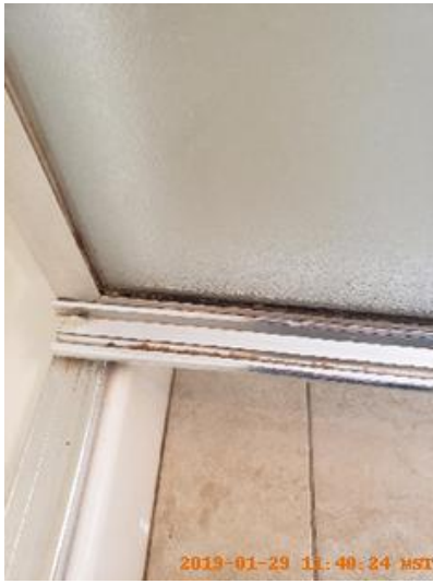
Shower Door/Rail/Curtain Taken on: 2019-01-29 11:40:24 Taken at: 43.56522778, -116.6039127 Image
